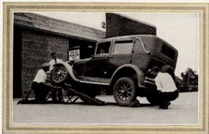
An unusual test of frame distortion
